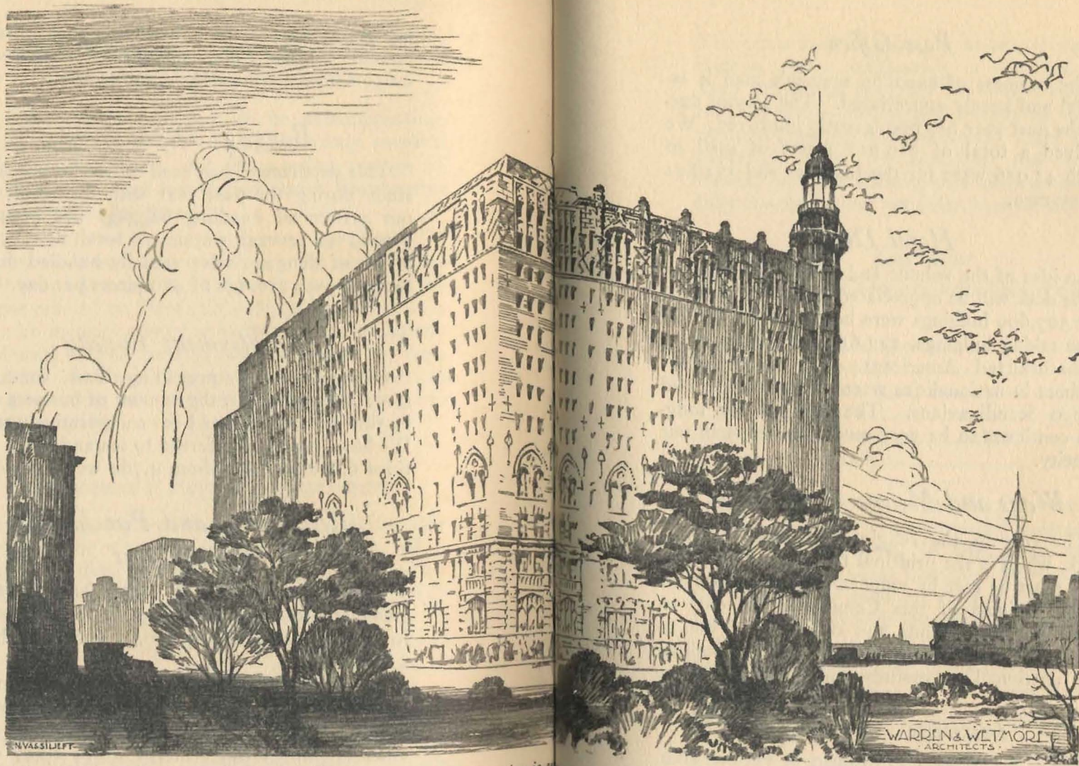
The Seamen's Church Institute with its annex, on which construction is in progress. Warren and Wetmore are the architects; John I. Downey, Inc., the builders. The present building faces South Street and runs along Coenties Slip. The Annex will have a frontage of 162 feet on Front Street and will occupy the space between Cuyler's Alley and Coenties Slip. It is fourteen stories high, with three basements, and will accommodate 1,500 men. When completed the Institute can provide 500,000 lodgings maximum. The present building is the shaded portion at the right.
