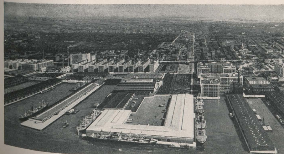
The terminal being built for the Mitsui Steamship Company at 39th Street, Brooklyn, will cost $10,600,000.
