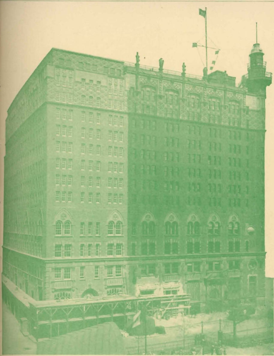
Present status of new Annex construction
