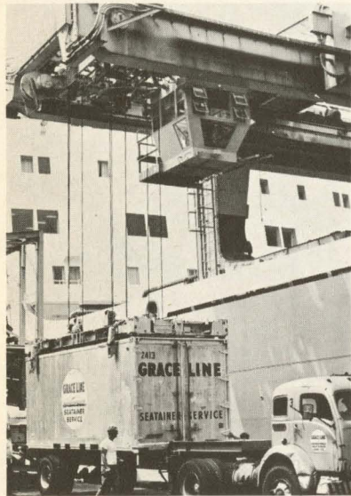
◀ Some of the newest container ships have their own built-in gantry cranes which are adaptable for operation on either the port or starboard sides of the ship.
