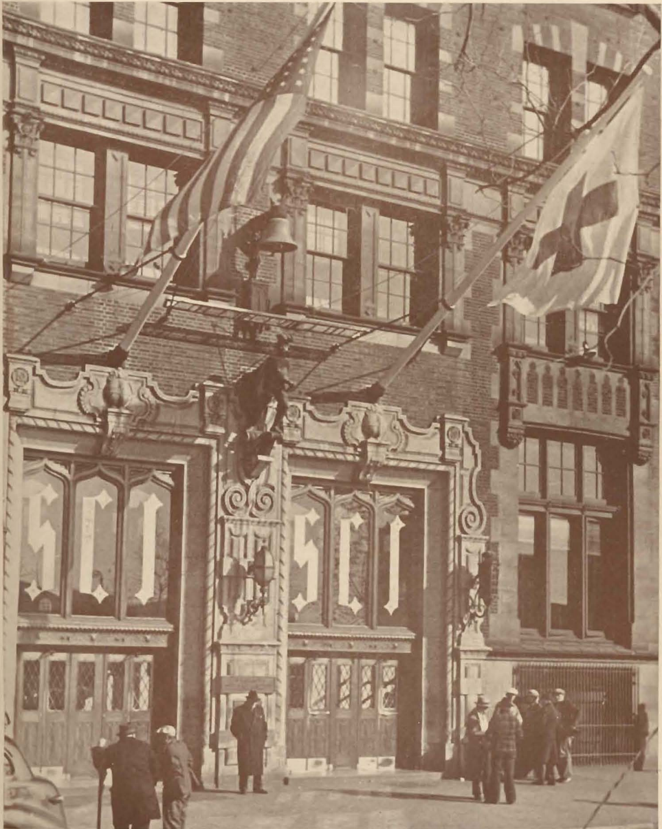
Main Entrance, 25 South Street
