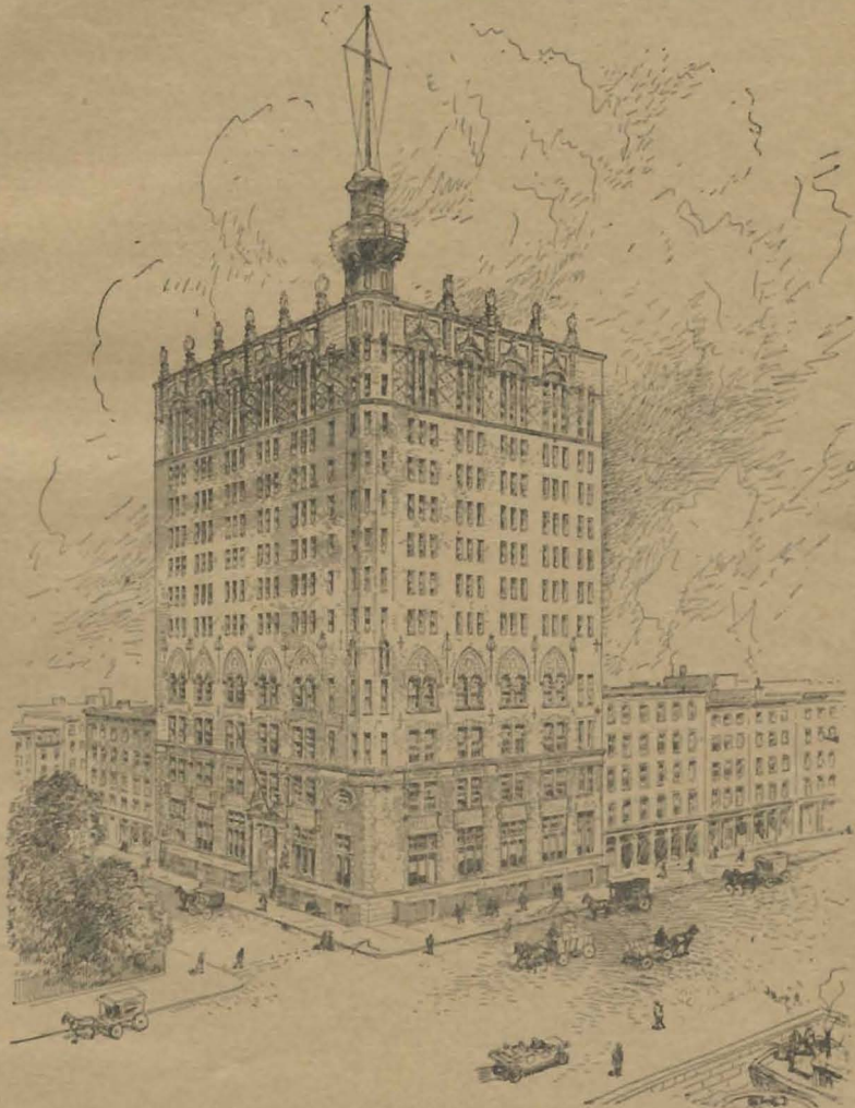
NEW BUILDING Now being erected
