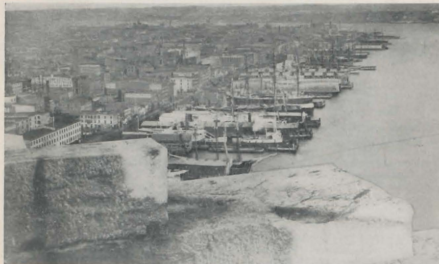
Photograph loaned by Robert F. Livingston A View of South Street, in the direction of Corlears Hook, from the partially completed Brooklyn Bridge, about 1876. The Institute's Third Floating Church is shown at the foot of Pike Street, close to the large full-rigged ship in the center of the picture.
